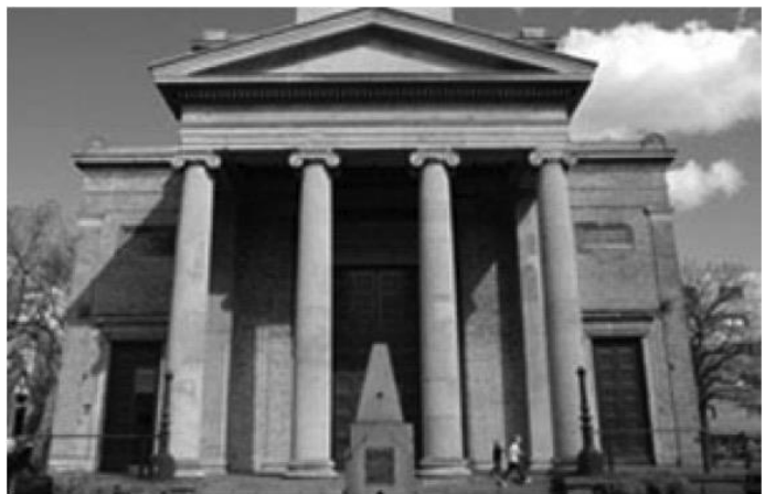
Location and vocation – some grand entrances: St James Church, Bermondsey (Home to the author's NHS surgery for nearly three decades)
